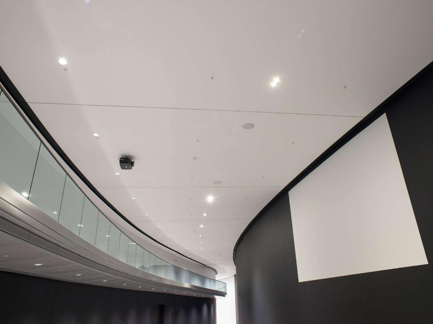
A long, sweeping tunnel links the Thought Leadership Centre with the rest of the campus. Throughout the tunnel McLaren required a flat black seamless surface interspersed with white squares on which to project film and images. Lucas laboratory technicians rose to the challenge and created new variants of our "Extraflex" coatings that flex and hold to the extremely long surfaces, and multi surface paints (MSP) to provide the reflective qualities required for clear moving images.
